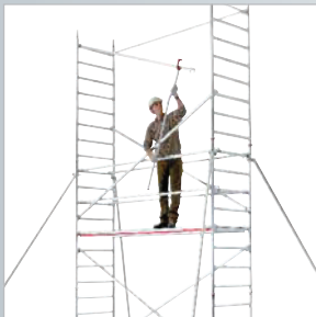
Hymer-Lifter during assembly
